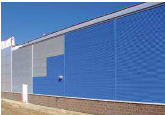
On a recent project, the Westbank Superstore, Tom Tar completed the entire building envelope.
