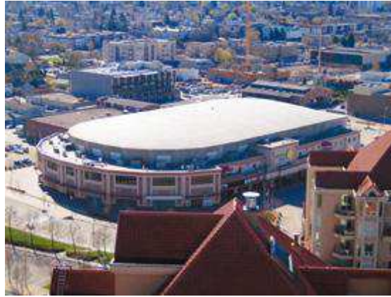
TomTar Roofing has completed an impressive number of commercial and industrial projects
