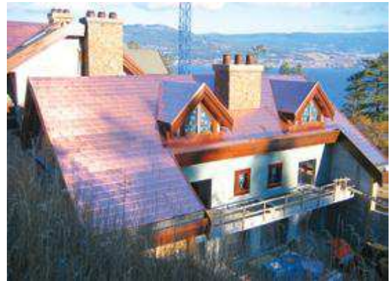
TomTar does exceptional work with copper roofing
